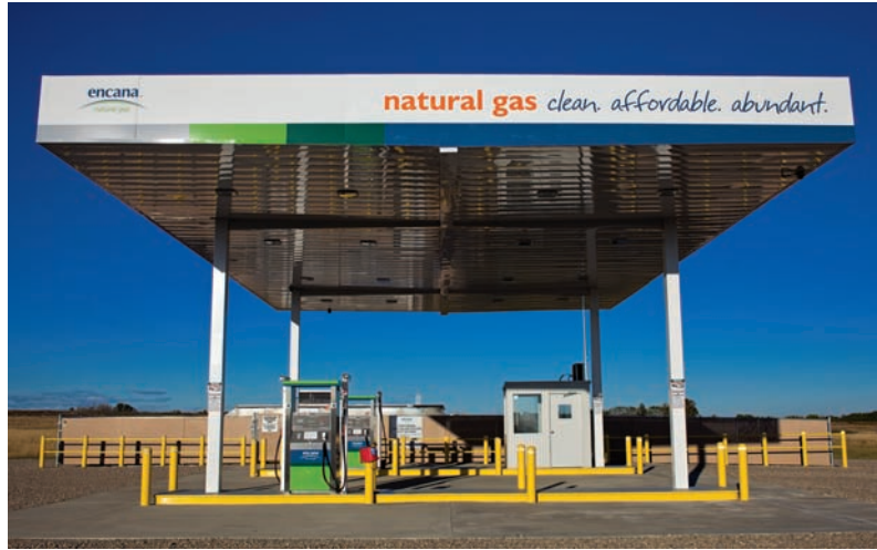
Encana's new natural gas fuelling station in Strathmore, Alberta.
